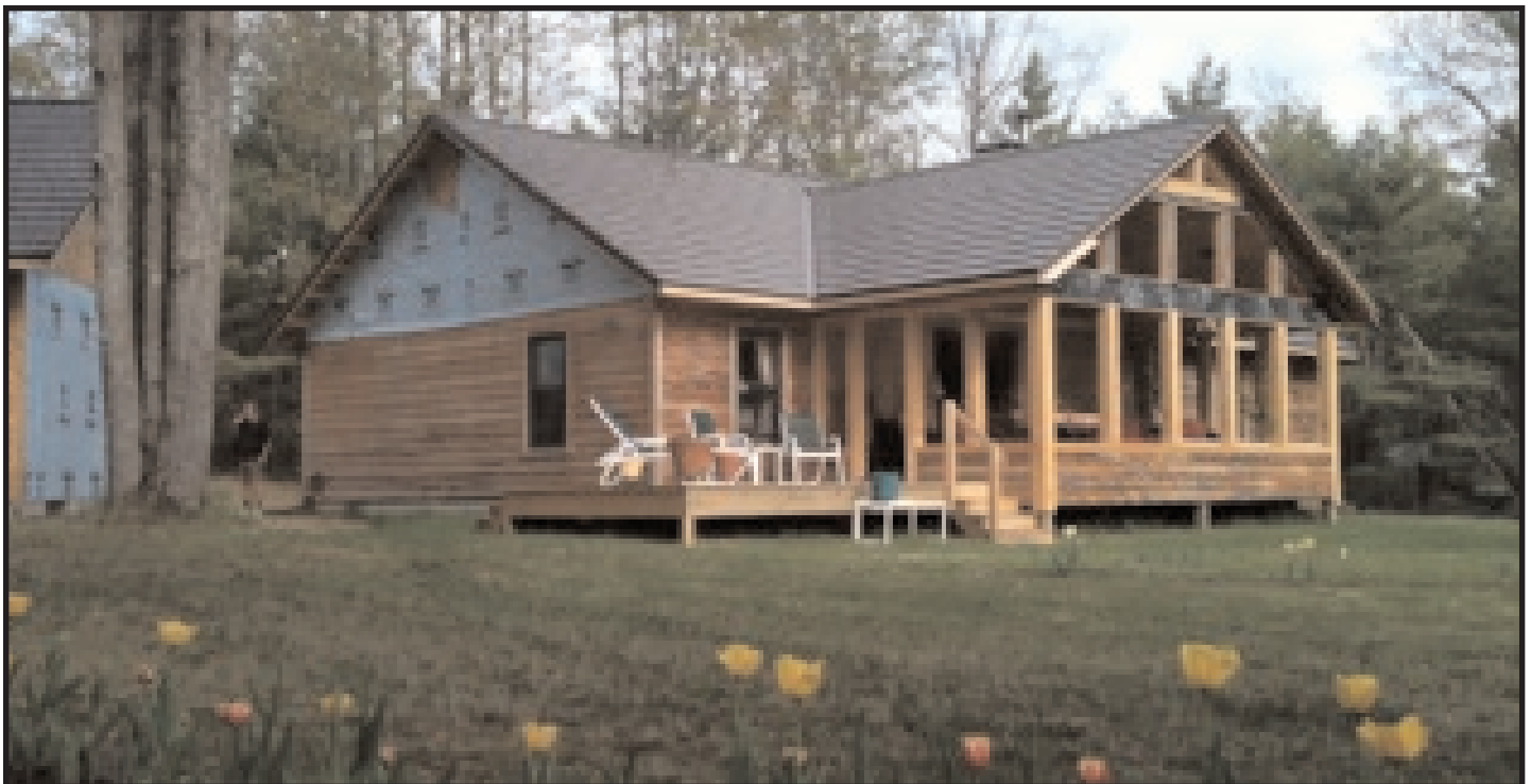
Karen Epperson is delighted with her new porch, deck and other improvements added to her home on Golden Lotus Trail.
